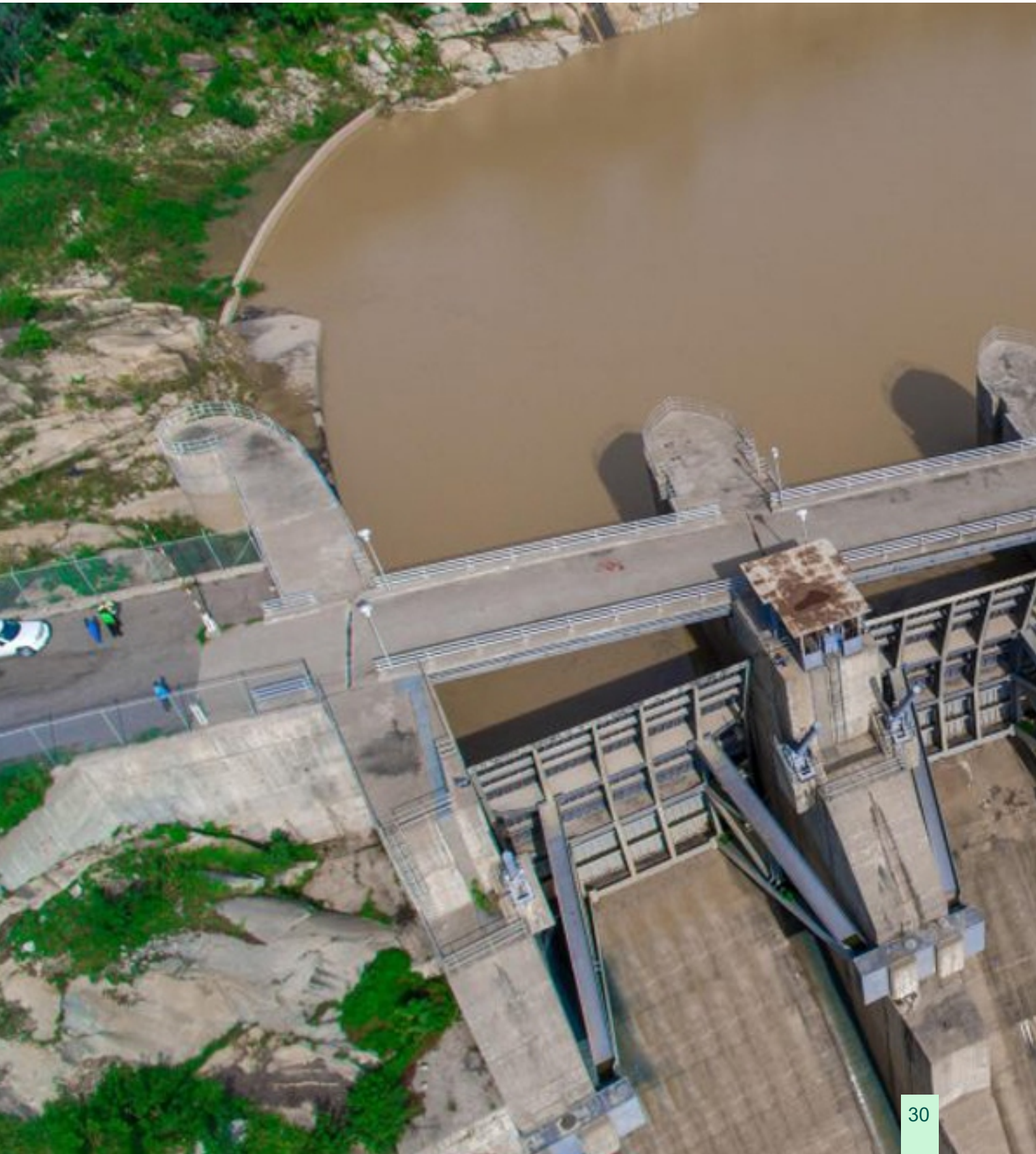
Figure 2 Kainiji Dam in Borgu Local Government
