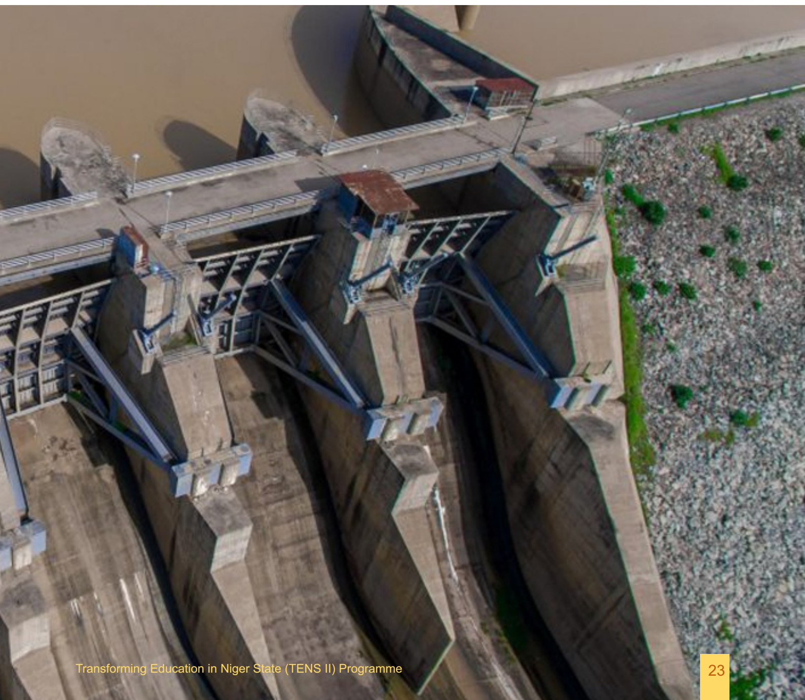
Figure 2 Kainiji Dam in Borgu Local Government
